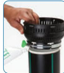
**6** To facilitate the assembly, it is recommended to use Huliote's pipe lubricant.
