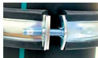
Upper sliding clamp tightening level
