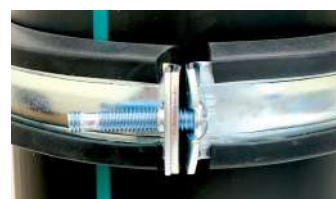
Lower Fixed clamp tightening level
